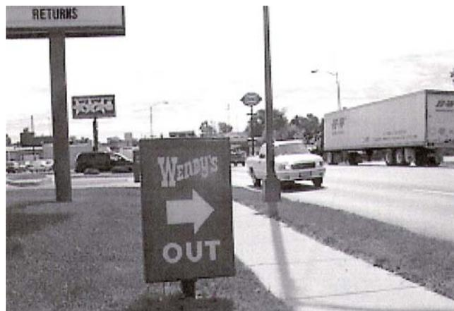
Figure 6 Inadequate site distance from a driveway
